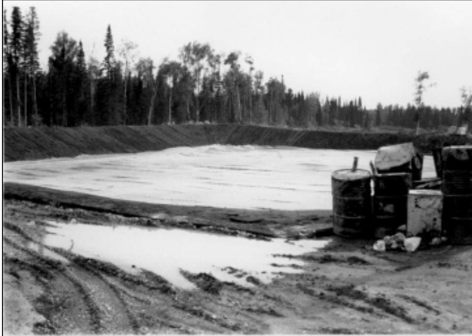
Final preparation of an interim landfill for solid hazardous waste in Tomsk oblast. The facility was built to mitigate the large volume of waste improperly stored at local enterprises while construction proceeds on the oblast's treatment facility. Photo: DJ Peterson.
