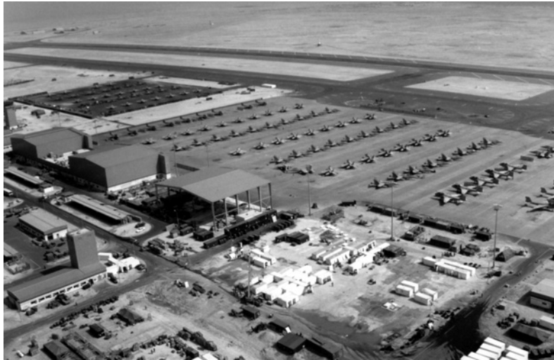
Figure 2.1—Parking Ramps at Shaikh Isa, Bahrain, Early 1991
