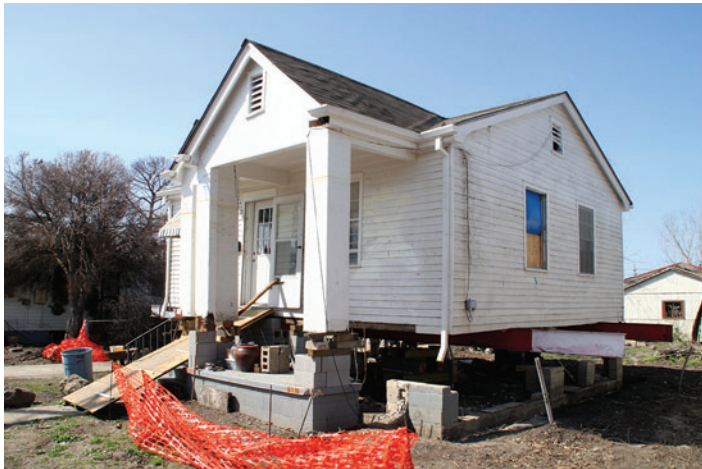
A home in the process of being retrofitted
