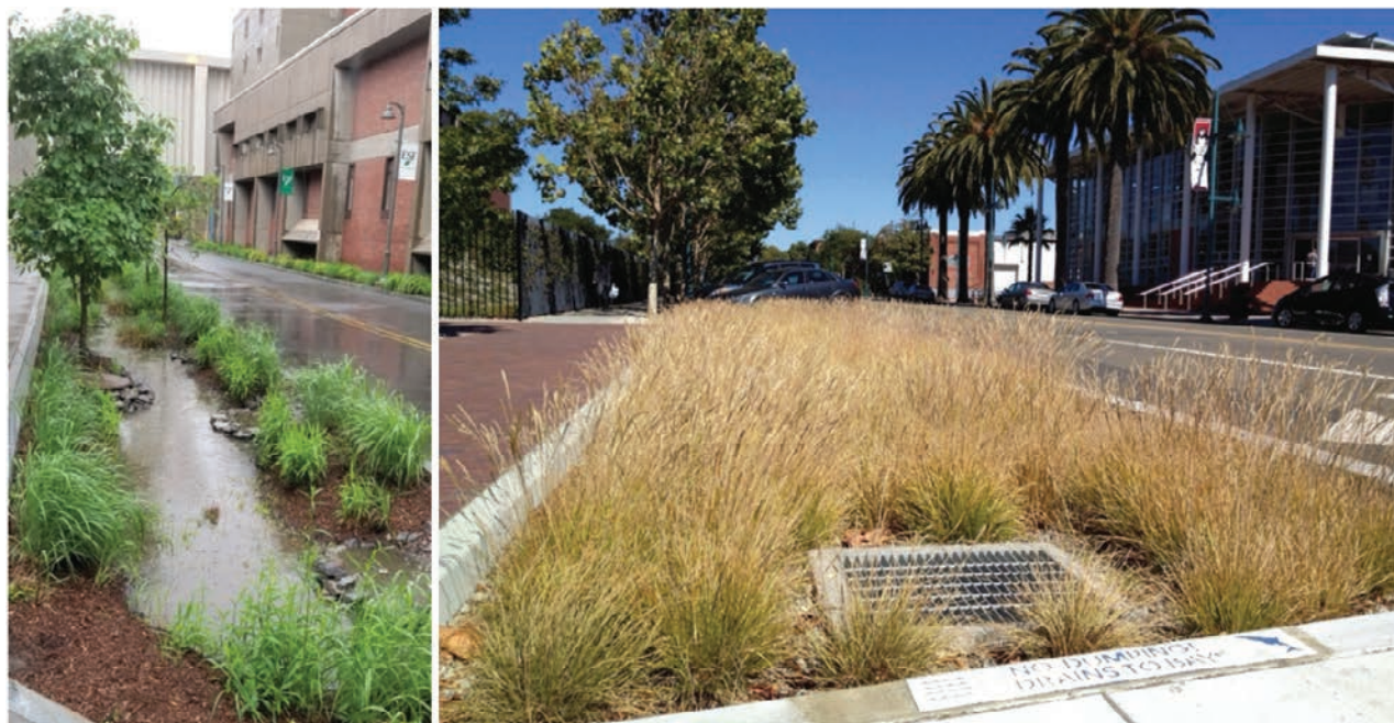
FIGURE 1 Examples of Green Stormwater Infrastructure
